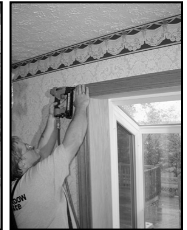
Install side casings & top section last, pin all corners
