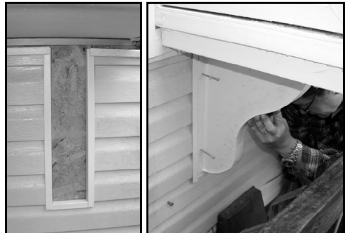
10. Prepare wall & attach braces to wall and bottom of seat
