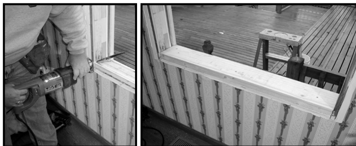
3. Remove window, cut out sloped sill, replace with flat sill
