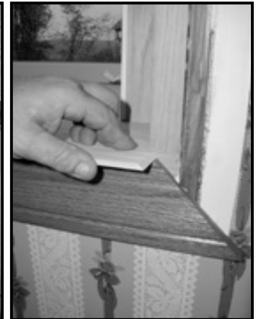
12. Cut & install bottom casing - *Note Reveal/Miter Guide
