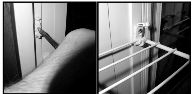
16. Insert Clip-Pin in hole, screw in place, wire shelf rests in clip
