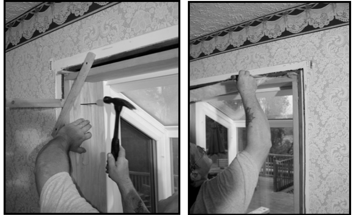
7. Secure frame in opening
