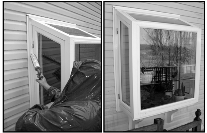
11. Seal all seams around the frame with silicone
