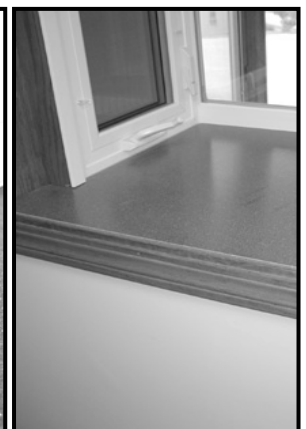
14. Slide Corian in place with good side up
