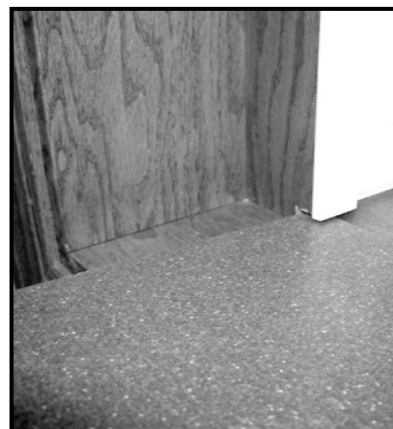
14. Slide Corian in place with good side up
