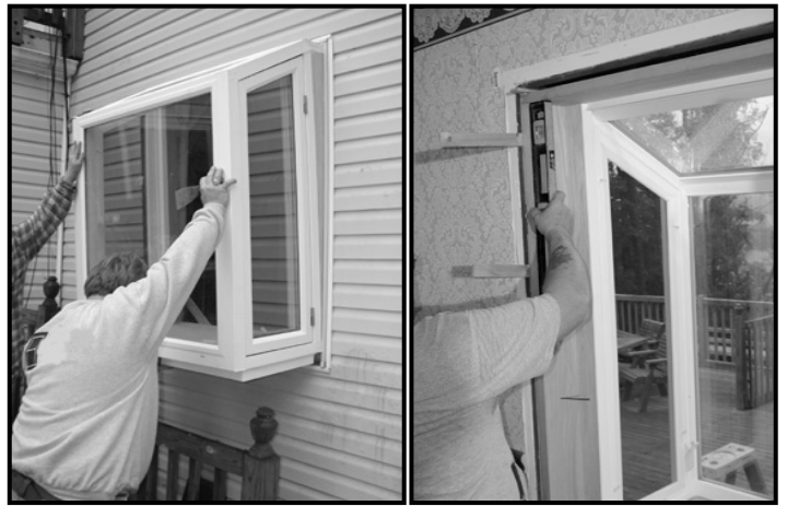
6. Slide frame into place, shim & level on all four sides
