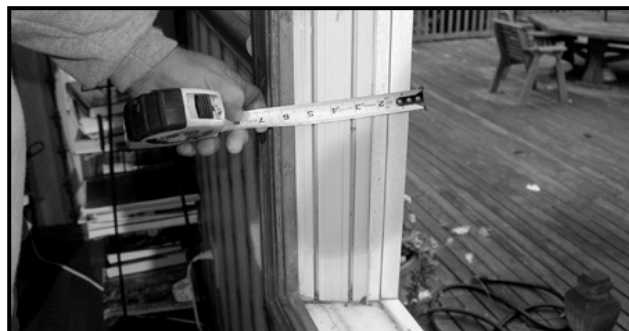
2. Jamb depth should equal the entire wall thickness
