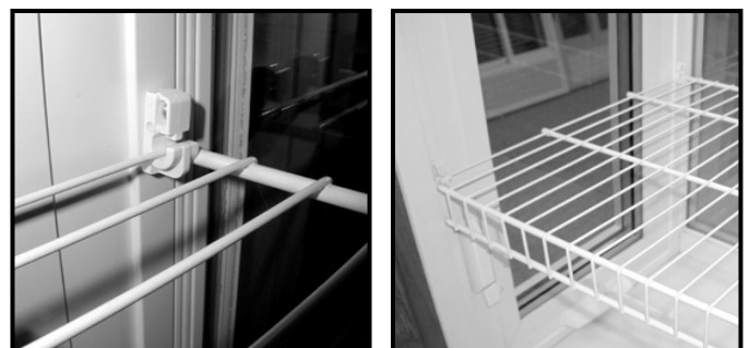
16. Push top down, snapping into place. Wire shelf is secure
