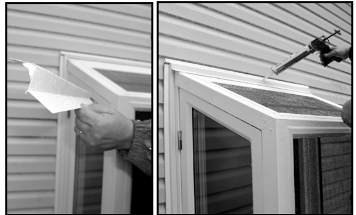
9. Install flashing and seal at top of garden window frame
