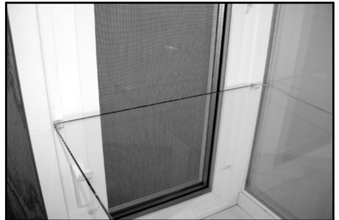
15. Glass shelf simply rests on the four holding pegs
