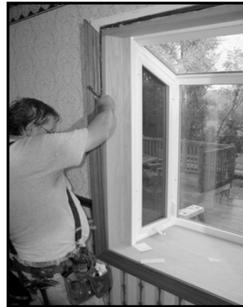
Install side casings & top section last, pin all corners
