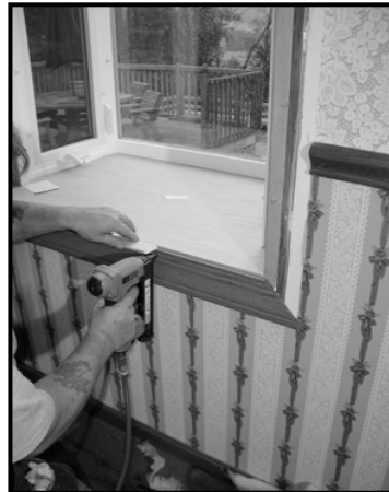
12. Cut & install bottom casing - *Note Reveal/Miter Guide
