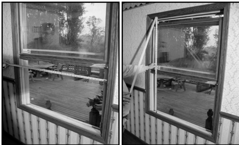
1. Double check all measurements prior to removing existing window
